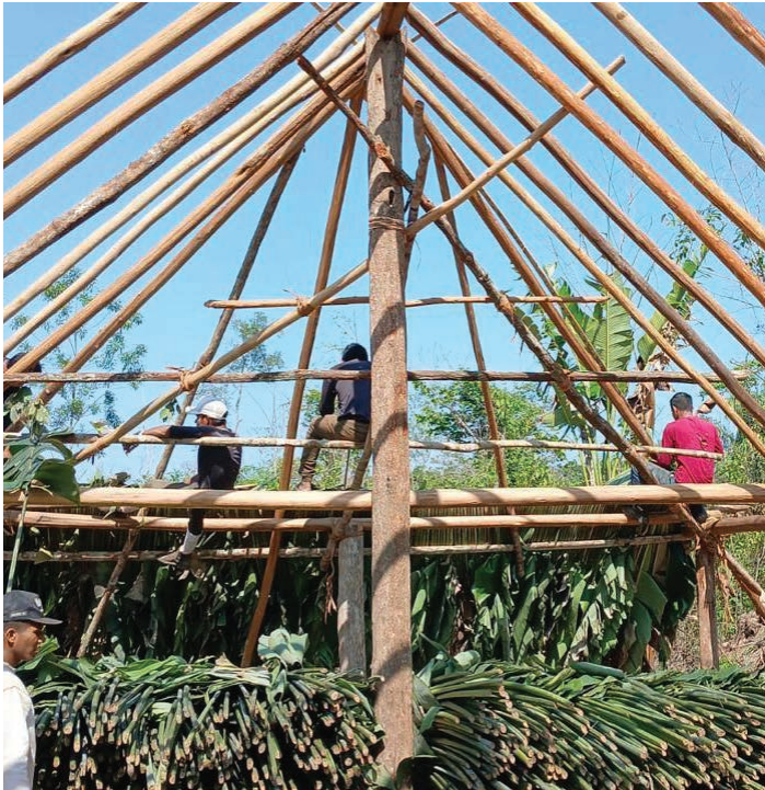
Constructing the new Capoto guard post in November 2025
